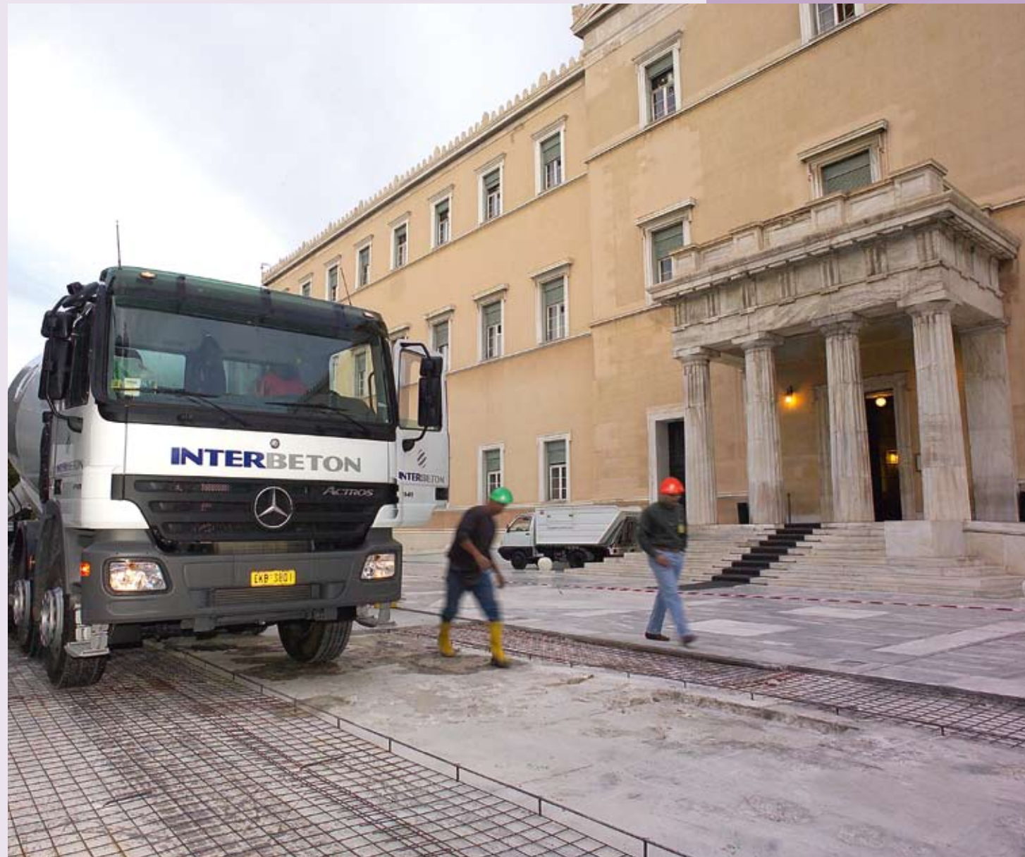
Application of new concrete products by INTERBETON at Greek Parliament
